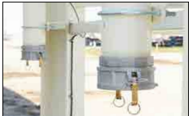
Fig 7 - Camlock couplers on fill tube ends
