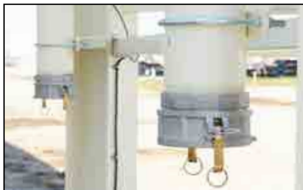
Fig 18 - Camlock couplers on fill tube ends
