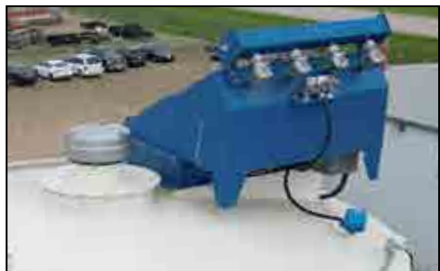
Fig 5 - Pressure relief valve and dust collector
