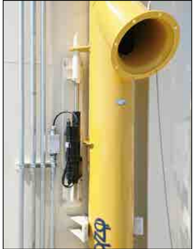
Fig 28 - Auger actuator and locking pin
