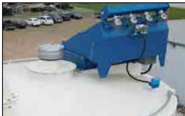
Fig 16 - Dust collector and pressure relief valve
